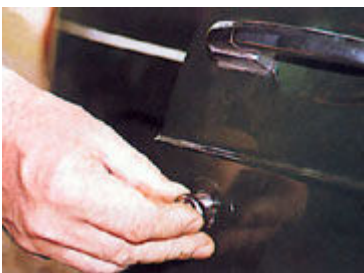
Pressing the new lock into place in the door skin.
