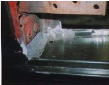
Separated joints turned back and rewelded with the seams sealed
