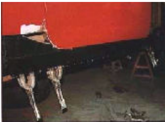
Bottom of outer sill clamped for welding
