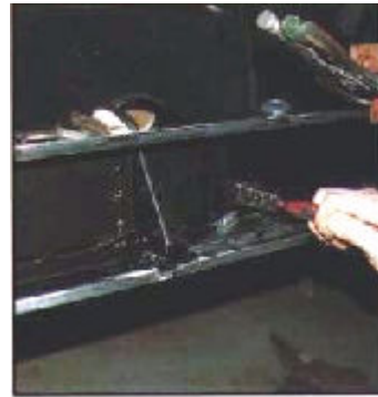
After welding apply rust proofing paint
