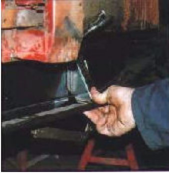
Using an extra jack reinforcing bracket to verify position and angle of castle section prior to welding
